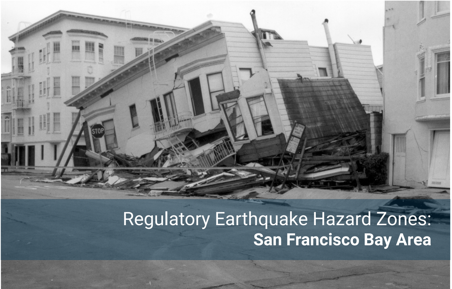
Damage to the Marina District from the 1989 Loma Prieta Earthquake. Photo: USGS
