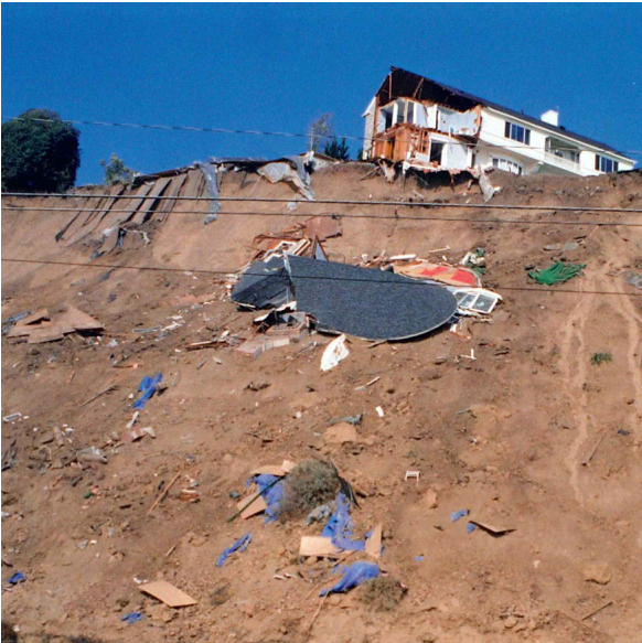
Landslide damage in Southern California. Photo: CGS
