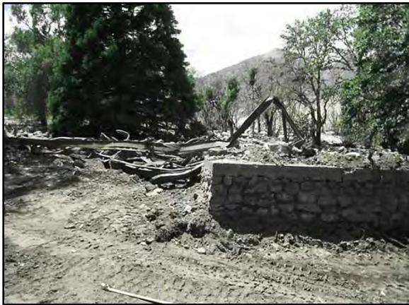
**Figure 25: Remains of the mobile home on the Bright Ranch. The twisted steel substructure of the mobile home lies behind the stone porch that was in front of the home.**
