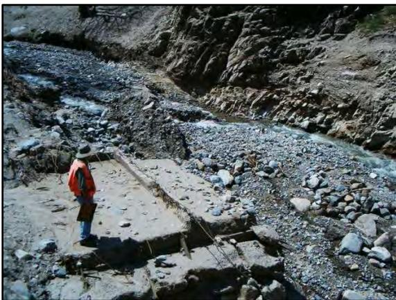
**Figure 26: Remains of the concrete abutment of the diversion structure on the South Fork of Oak Creek that was partially swept away by the debris flow.**
