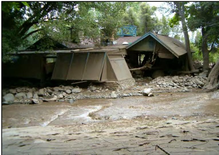
Figure 34: This home was damaged by boulders while others were damaged mostly by finer grained sediment. The water in the foreground is from Oak Creek which was forced from its channel during the storm. It was restored to its original channel (Locality 16, on Figure 33) soon after the storm, so residents could access their homes (Photo by Jim Stroh).
