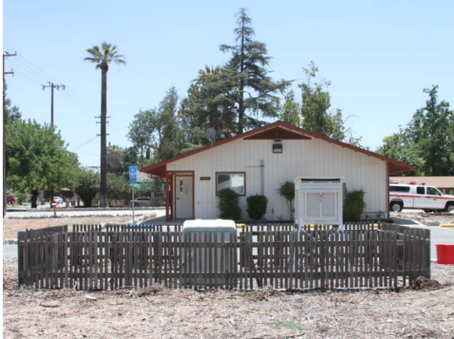
Looking south from array 12102-1 towards enclosure housing CE.12673 seismic station and fire station housing CE.12102 seismic station
