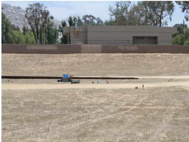
Looking northeast towards fire station from passive surface wave array 13080-1
