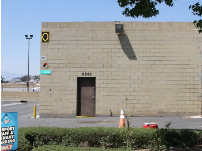
Looking north towards building housing CE.13123 seismic station from HVSr Location 1
