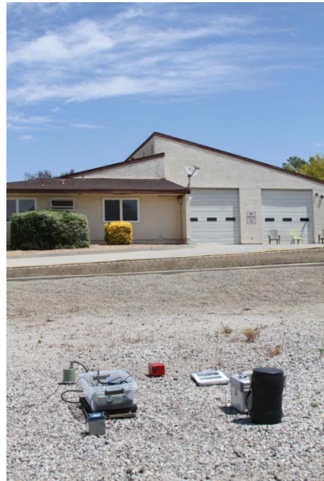
Looking north towards fire station from HVSr Location 1
