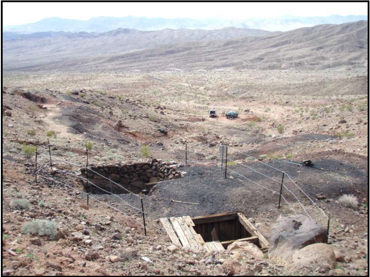
Fencing installed around hazardous mine shafts on State land in San Bernardino County. Photo: DOC (2015)
